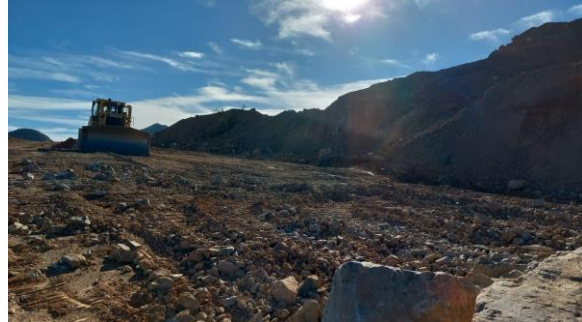
Ground pads ready at the Avino property
