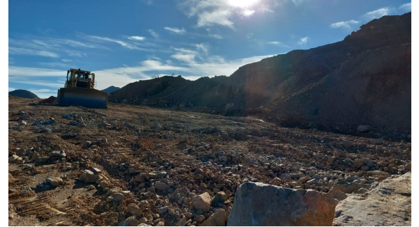
Ground pads ready at the Avino property
